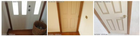
Striker plates to the doors within some rooms need minor adjustment to ensure the doors secure correctly when closed. A licensed carpenter is required to provide a further assessment and to offer suitable rectification as required.
