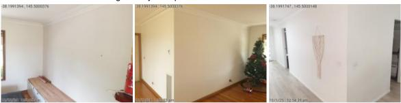
Minor cosmetic settlement cracks were noted to the wall lining within some rooms. Minor cracking can be expected in the type of lining. However, maintenance is required by a suitably qualified plasterer to repair the cracking present.
