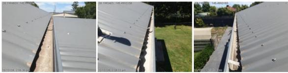
Some downpipes to the rear elevations do not appear to be connected to a stormwater dispersal system. These should be connected without delay to prevent decay to surrounding components and to prevent the foundations of the dwelling being damaged. This also effects the timber pest management of the property and may attract termites. A licensed roof plumber is required to provide a further assessment and to offer suitable rectification as required.
