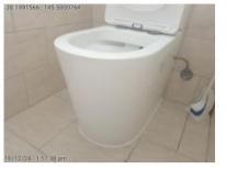
However a leak is present at the rear of the toilet pan and appears to be caused from either a leaking pan/waste seal or cistern leak. This needs to be repaired to prevent decay to surrounding components. A licensed plumber is required to provide a further assessment and to offer suitable rectification as required.
