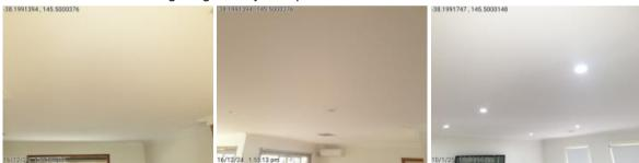
Evidence suggests there is past or present leaks to the ceiling lining within the hallway. No leaks were visible on the day and moisture readings were normal, suggesting that past leaks may have been repaired. However further investigation is recommended to ensure no current leaks exist and to prevent potential structural decay. A licensed builder is required to provide a further assessment and to offer suitable rectification as required.
