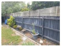
However a section of the fences on the south boundary are generally in poor condition. Severe wet rot decay, and other defects were noted to these timber fences and decayed timber needs replacement by a carpenter.
