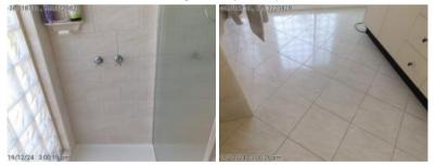
A flexible sealant should be re-installed by a suitably qualified professional to the gaps between tiled walls & base of the shower. This is to prevent water penetration and decay to surrounding components.
