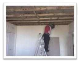
A false ceiling can often be discovered when accessing the roof space a simple measurement can be taken of the ceiling height at the access hatch and applied to other rooms for comparison.
