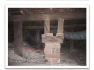
Older houses often require re-stumping. In most cases in older houses red gum timber was used for stumps, and while it was a durable material, it's life span was only around 60 -80 years. This means that any house that has the original red gum timber stumps may be requiring the stumps to be replaced.
