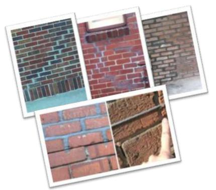
Often brickwork above the floor level in houses is non-structural, however when brickwork cracks it is vital that a diagnoses of why it has occurred is undertaken. In most cases it is impossible to fix without removing the brickwork and starting again, so when it is observed that brickwork has been patched or remortared it may be covering-up larger structural footing or foundation issues that could be costly.
