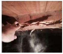
If the joists and bearers are rotten or damaged they may need to be replaced, and the moisture problems that caused the decay should be addressed. Assuming the joists are in good condition, the solution to both sagging and bounciness problems is to reinforce the floor by either beefing up the floor joists or adding new posts and/or a new or reinforced support beam where this is practical. Either way if floors are springy, it's important to establish the cause prior to purchase.
